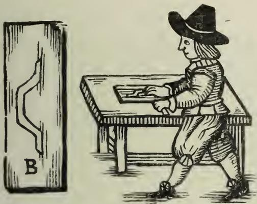
FIG. 1. MAKING THE COFFINS OF PAPER (ROCKET-CASES). (RICH CABINET, 1677.)
